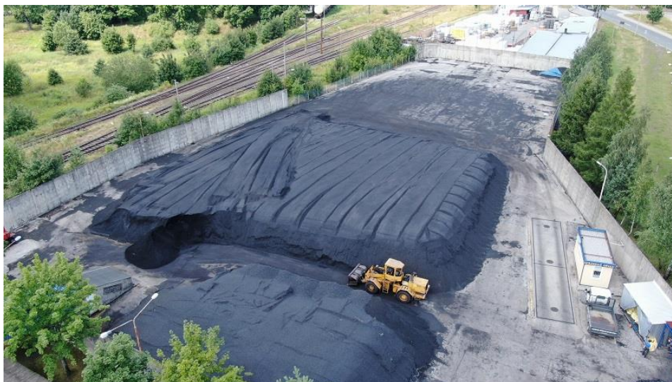
Figure 2-81. View of the carbon park
