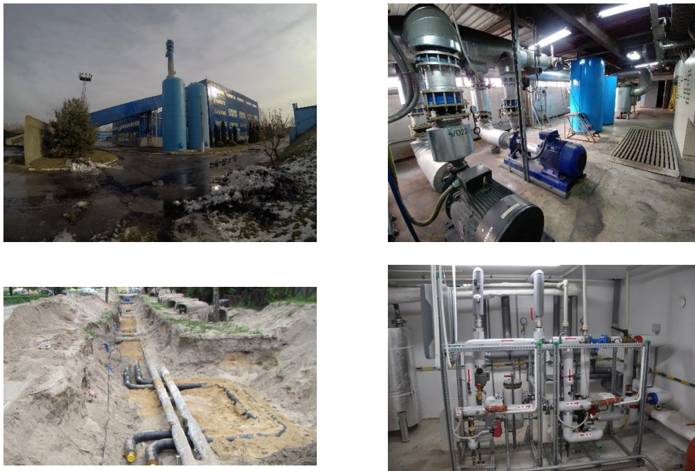
Figure 2-55. Żyrardów District Heating installation
