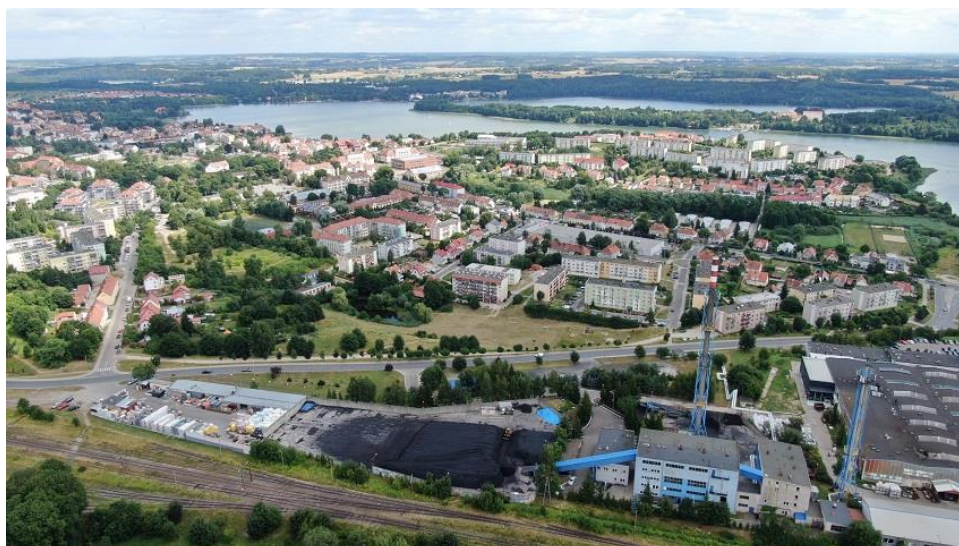
Figure 2-78. View of the Mrągowo municipality with the coal boiler facility on the front 40
