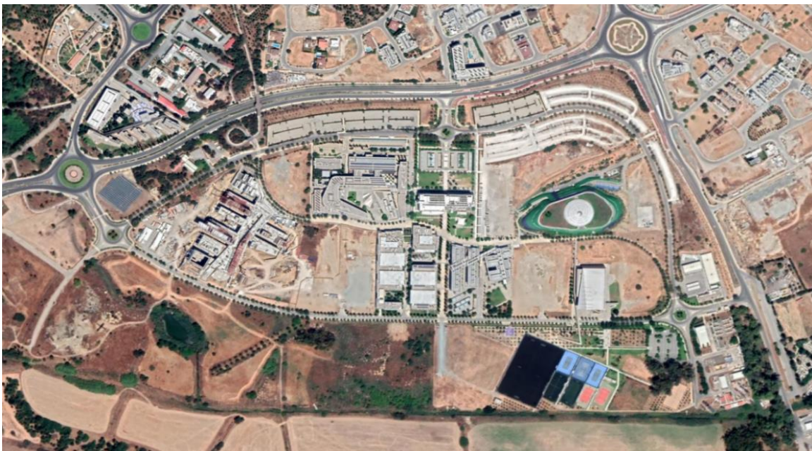
Figure 2-42. University of Cyprus – Aerial campus photograph.
